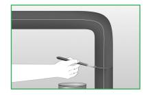
Seal all joints with Armaflex Adhesive. **Do not stretch when sealing joints.**
