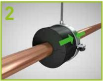
Close the seam applying firm pressure. Push the pipe support into the open clamp. It must be in the middle of the clamp.
