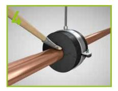
Before insulating the pipe, glue the edges of the pipe support to the pipe.
