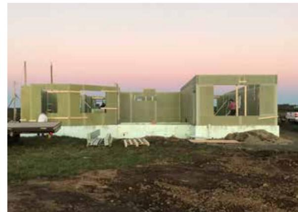
©JD Composites: Eco-House consists of 170 ArmaForm cored SIPs, assembled in 14 hours.
