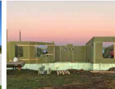
// Eco-friendly house in Nova Scotia, Canada. The 186 square metres prototype bungalow consists of 170 ArmaPET cored SIPs and was assembled in just 14 hours. 612,000 recycled PET bottles brought this eco house to life.
