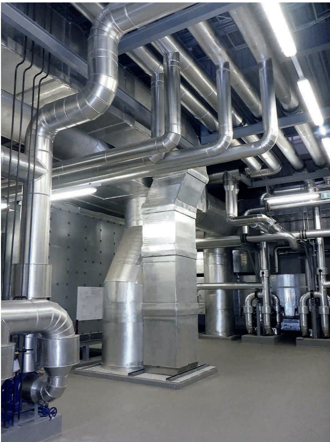
The seams were secured with the Arma-Chek Silver self-adhesive tape
