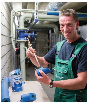
The new insulation material made by Armacell can be cut neatly and glued easily.
