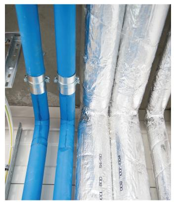
Armaflex Ultima not only protects the pipes against condensation and unnecessary energy losses, in a fire it develops 10 times less smoke than traditional elastomeric insulation materials
