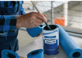
For installing Armaflex Ultima, Armacell provides adhesives which have been specially developed for use with the new Armaprene® insulation materials, such as Armaflex Ultima 700 adhesive
