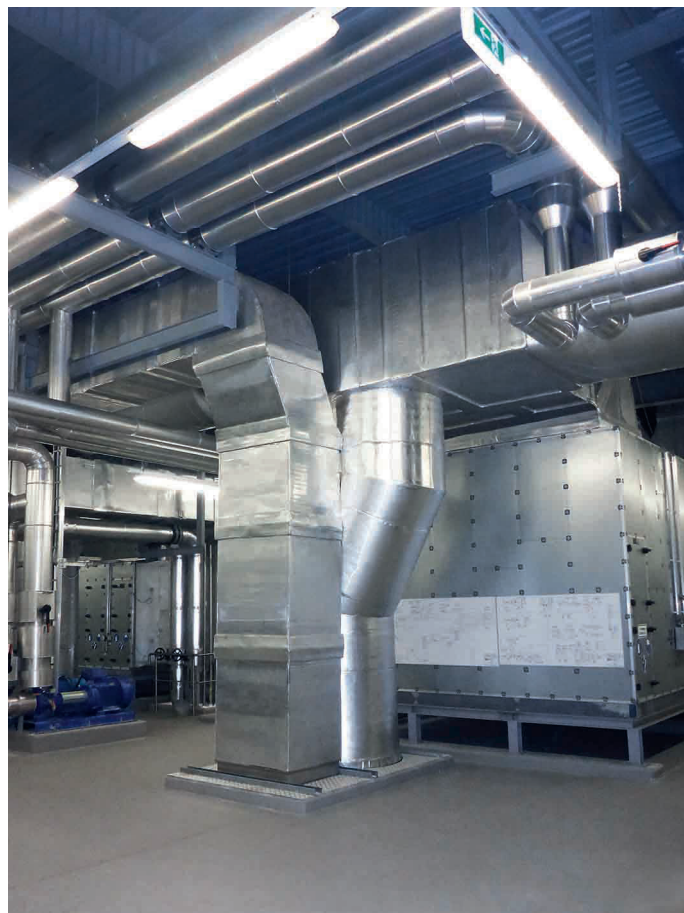
The central air-handling station is located on a separate floor under the roof of the new building
