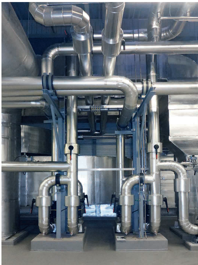
The ventilation installations were insulated with around 10,500 m 2 of Arma-Chek Silver sheet material
