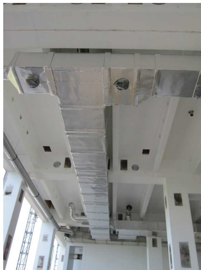
The air-ducts in the production hall are exposed to very high temperatures and 70 % humidity
