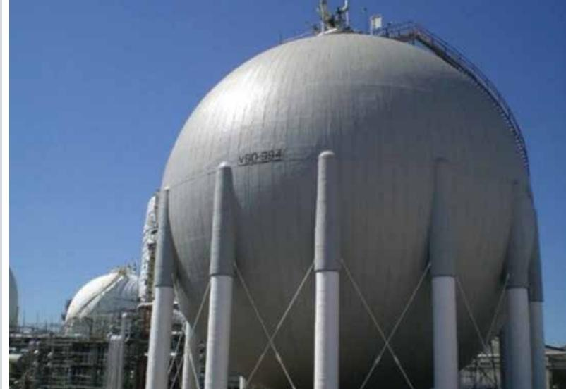
and its contents. It was critical that whatever product was chosen to insulate the tank didn't interfere with the reaction of the fireproofing in the event of a fire. Shell ordered the coatings manufacturer to perform high temperature burn tests at their R&D facility in the UK.
