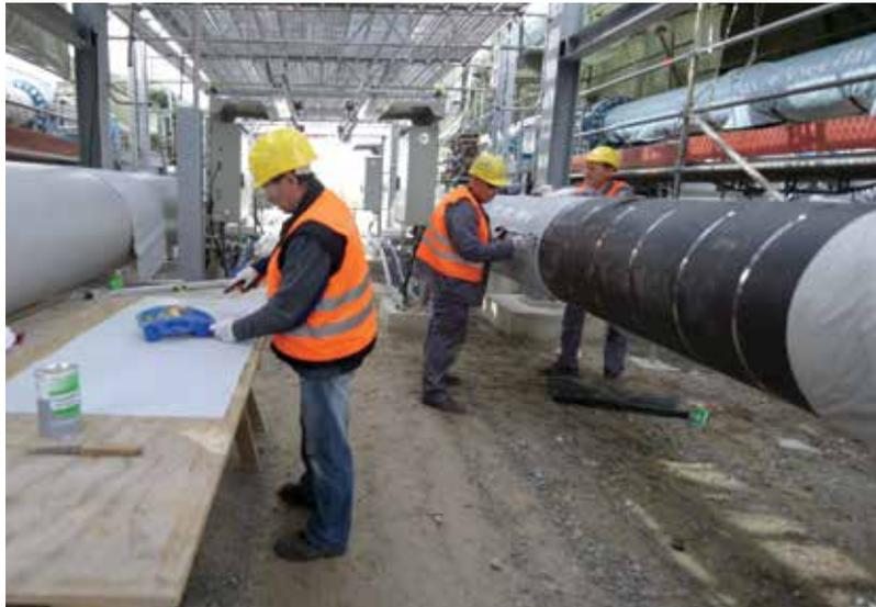
insulation constructions, ArmaSound Industrial Systems meet the noise-control requirements with reduced insulation thickness and weight.
