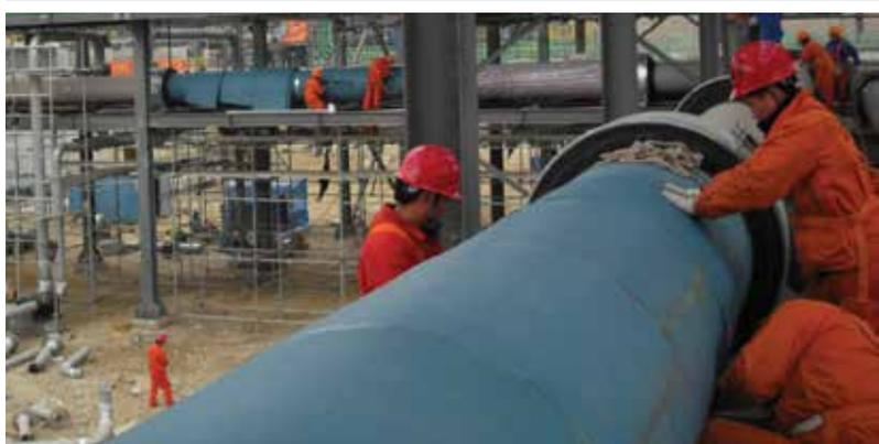
The LNG process pipework was insulated with the multilayer Armaflex Cryogenic System.
