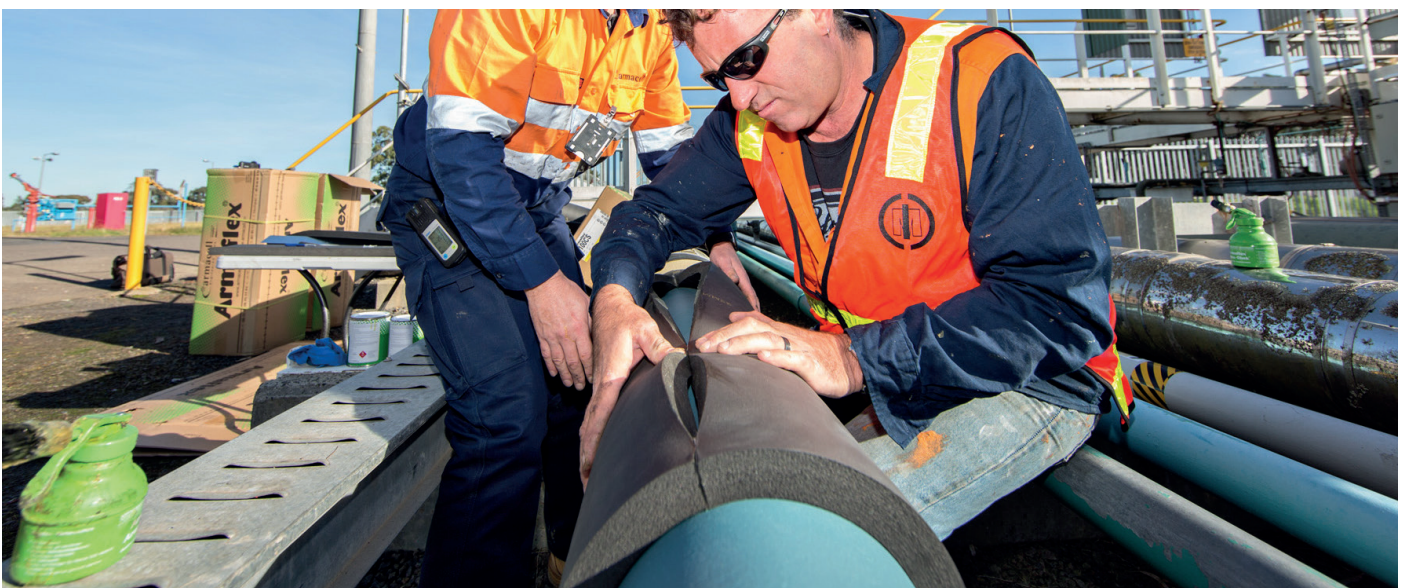
The multi-layered Armaflex Cryogenic Systems ensure exceptional thermal insulation, reduce the risk of corrosion under insulation (CUI) and allow considerable cost savings during the installation process
