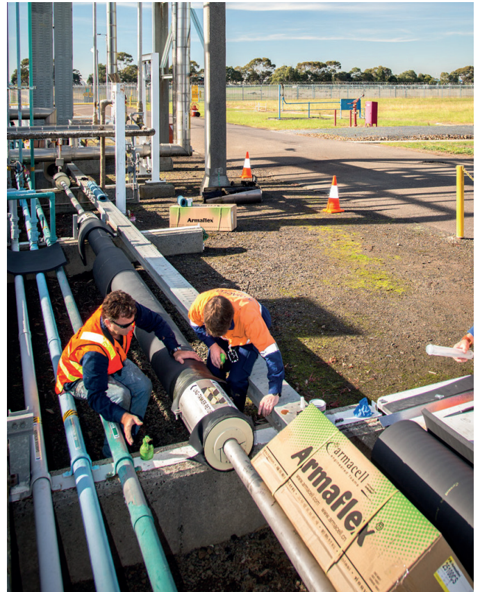
The insulators from Insulmet Pty Ltd (Moe) received training in the application of the new Armaflex Cryogenic Systems from Armacell
