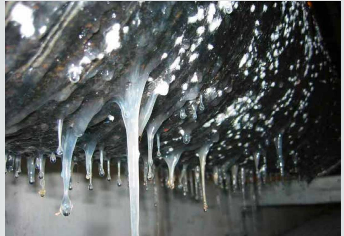
It should not look like this: insulation which works well at first, but on which condensation or – as here – even ice forms after the equipment has been in operation for a while
