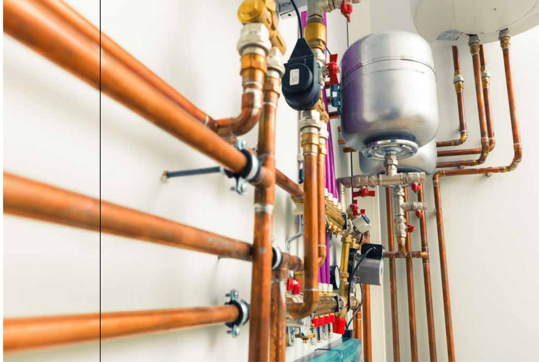
The annual heat loss due to uninsulated distribution pipes and fittings in the cellar can account for up to a quarter of the yearly heating energy consumption
