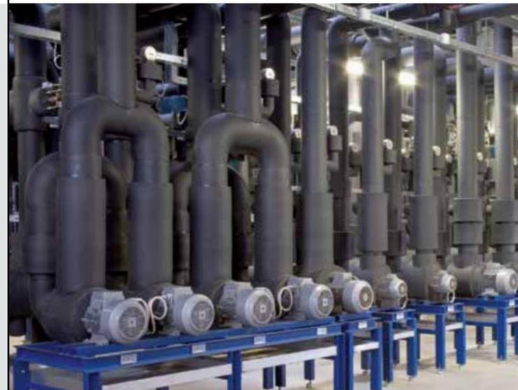
As a study by Ecofys, a leading international consultancy in the field of renewable energies and energy efficiency, shows, insulation of industrial plant is not usually economically designed. By installing optimized insulation systems, it is possible to achieve energy savings of up to 45 %. The investments have often paid off after just a few months. Unlike for the building or transport sector, there are as yet no corresponding legal regulations or energy-saving programmes for industry.
