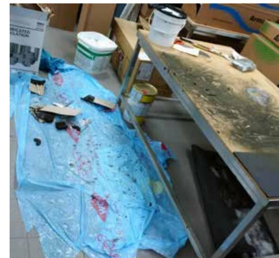
When installing PUR and cellular glass, considerable amounts of dust occur and the working area must always be covered with a tarpaulin.
