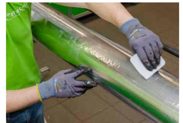
PUR is also glued using a two-component adhesive. Then an aluminium adhesive tape must be applied on all longitudinal and circumferential seams to create a diffusion-tight seal.
