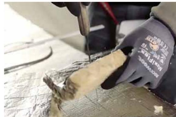
The manufacturer's application video shows just how easy it is to damage the vapour barrier: while cutting out a piece for a component, the insulator pierces the mat underneath without noticing it. Even such small defects are enough to prevent the vapour barrier working effectively.
