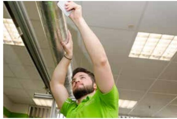
Mineral wool pipe sections are fastened with an overlapping self-adhesive strip and the join is then smoothed using a spatula. For additional security, aluminium tape is wrapped around the pipe sections at least every 600 mm.
