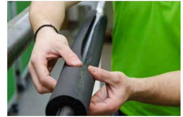
Elastomeric insulation materials are available as standard and self-adhesive products. After applying adhesive or removing the protective foil the edges are simply pressed together section by section. No further measures are needed to secure the seam.
