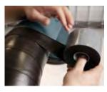
around the insulated pipe with an overlap of 20 mm. The self-welding material
