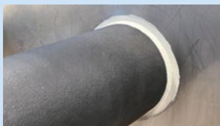
To prevent flames and smoke from spreading in the event of fire, firestop penetrations through bulkheads and decks must be professionally sealed off. By combining the proven properties of ArmaFlex with an intumescent component, ArmaFlex Protect guarantees reliable fire safety in all A-class division and B-class bulkheads without the need for any complicated additional measures. At the same time, this product ensures effective thermal insulation and reliable condensation control.
