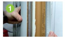
Open the pipe shell and place around the pipe which is to be insulated.
