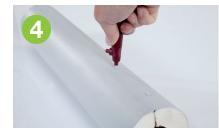
Alternatively, the overlap of the longitudinal seam should be fastened with rivets. At ambient temperatures above +40 °C and on pipes which will not be accessible later, the seam should be additionally secured with plastic rivets (at least 5 per metre).
