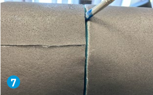
7 Apply adhesive onto the circumferential seams.
