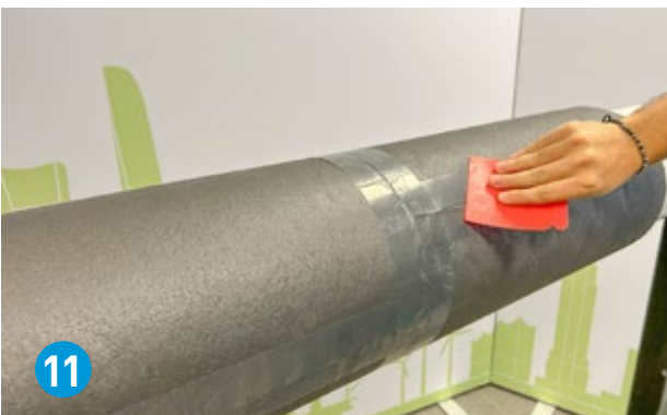
11 Use a plastic spatula to smooth the ArmaFlex Ultima C tape surface.
