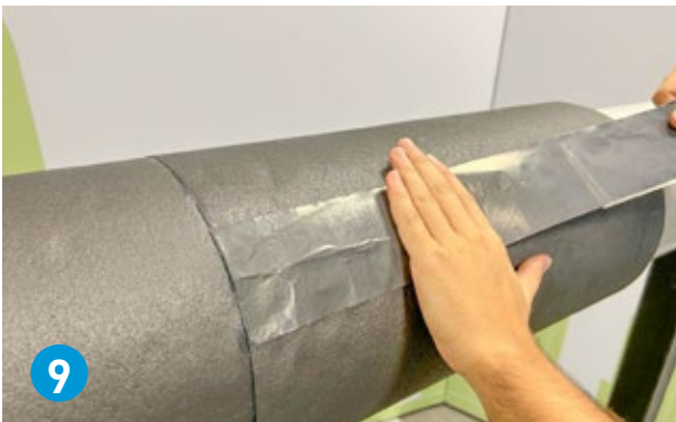
9 Apply ArmaFlex Ultima C tape on the longitudinal seams.
