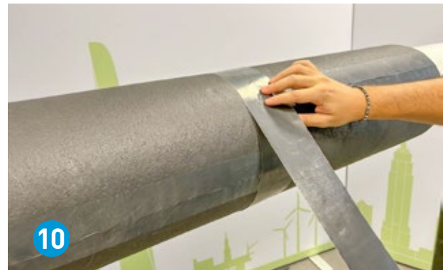
10 Apply ArmaFlex Ultima C tape on the circumferential seams.
