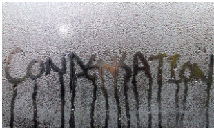
Condensation/ sweat control
